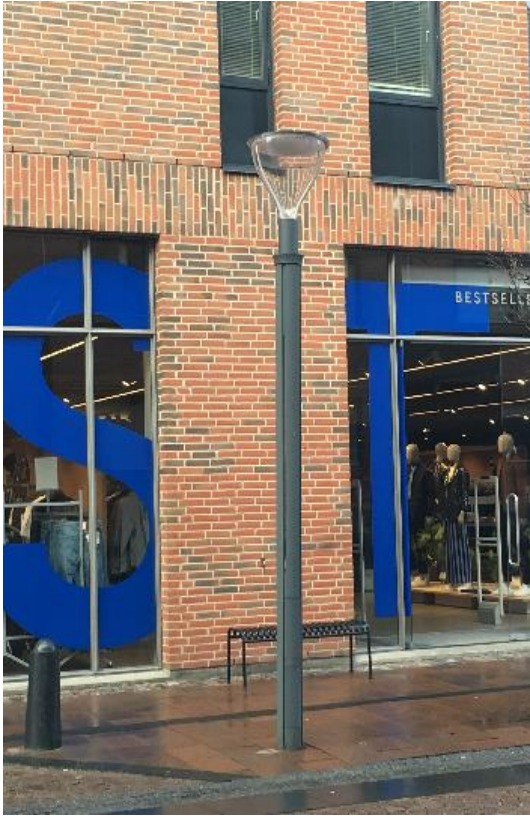
Figur 2 - Nyt gadelysarmatur (Philips Metronomis LED)
